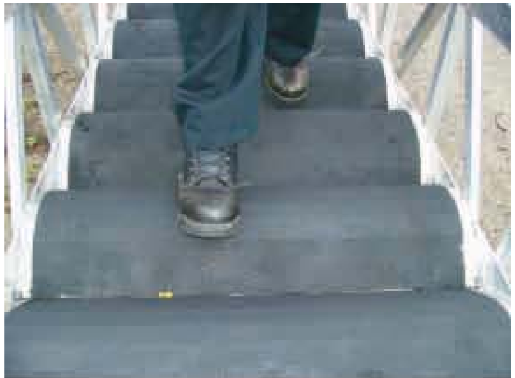
Slip resistant curved tread walk surface
